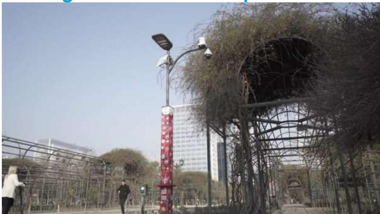
In 2019 Infinet Wireless' smart security and connectivity technology was deployed in the Las Condes community in Santiago, improving safety for the residents. The more than 110 smart posts feature strategic interconnection points for the complete monitoring of zones (squares), panic buttons, Wi-Fi and PTZ cameras for the citizens' security.
